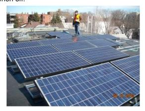
FACT: 95-97 Pine Street has 50 Solar Photovoltaic Panels that use the sun's power to generate electricity for hallway and basement lighting.
